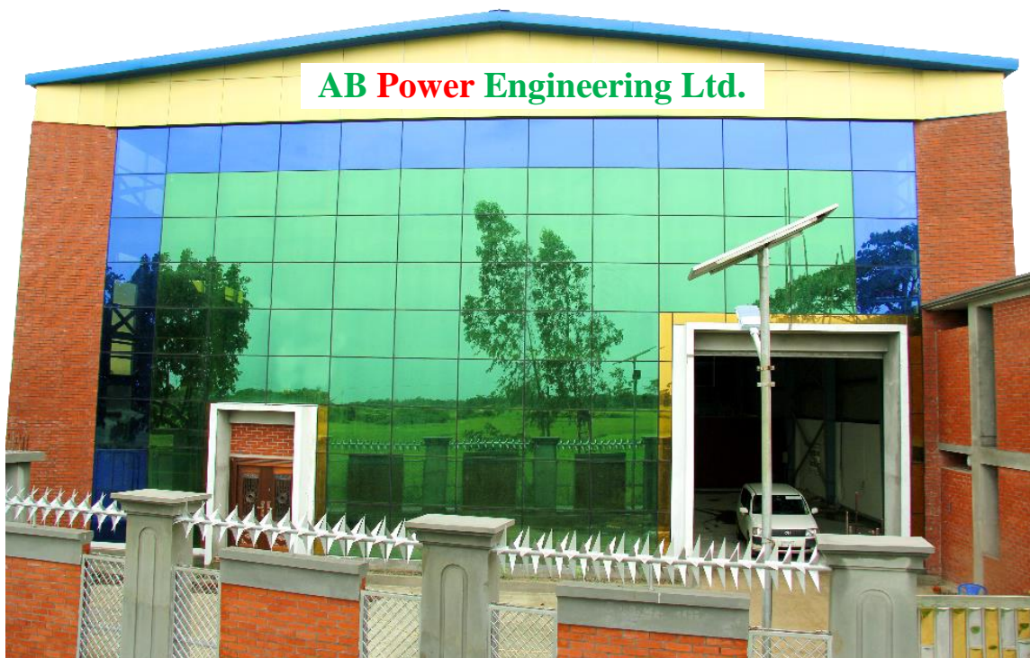
Factory of AB Power Engineering Ltd.
